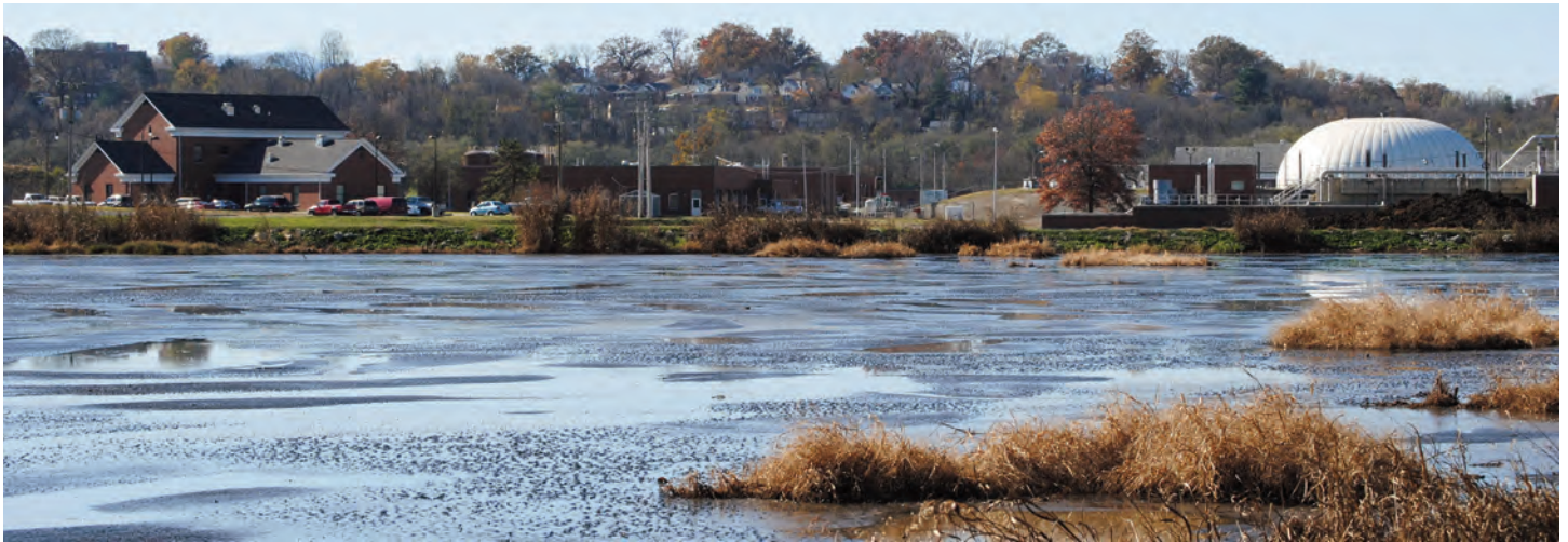
The treatment ponds at the Western Virginia Water Authority's water pollution control plant are a preferred bird watching site in Roanoke.
