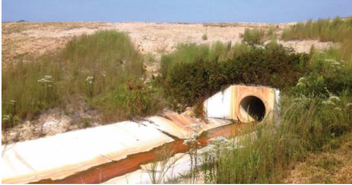
Acid sulfate runoff can damage concrete and metal and affect local water quality. Note the brown water and stains on the concrete.
