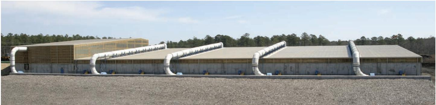
McGill-Sussex plant is the largest enclosed composting facility in Virginia. Biofilter (foreground) removes odors and particulates from plant exhaust.
